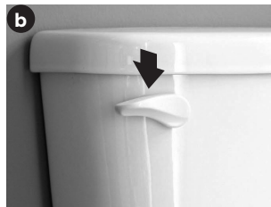
Flush the toilet to drain the tank. Use towel or sponge to remove remaining water.
