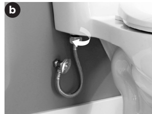
Loosen the nut "counterclockwise" by hand and remove the supply hose. If tools are needed to remove the nut, please replace the supply hose with a new one when reinstalling.
