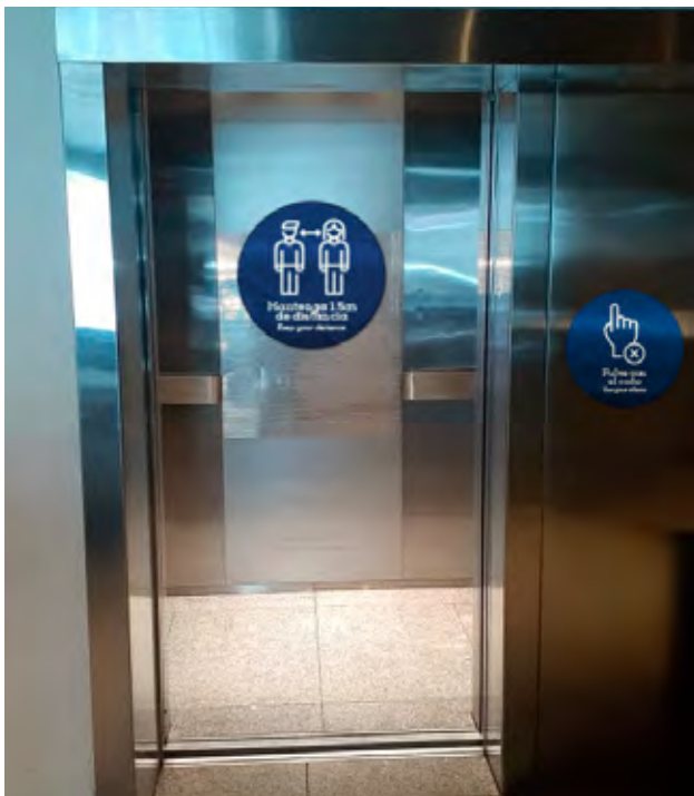
Push-button panels and elevator entrance.
