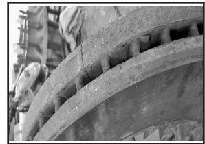
Unacceptable Crack FIGURE 108
