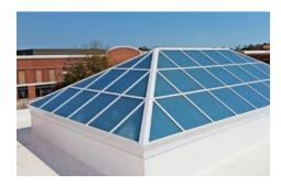
Gloss powder coat finish formulated with durable fluoropolymer resins and solar-reflective pigments.
